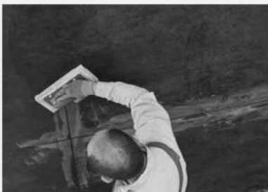
fig.39 Fugowanie / Grouting.
